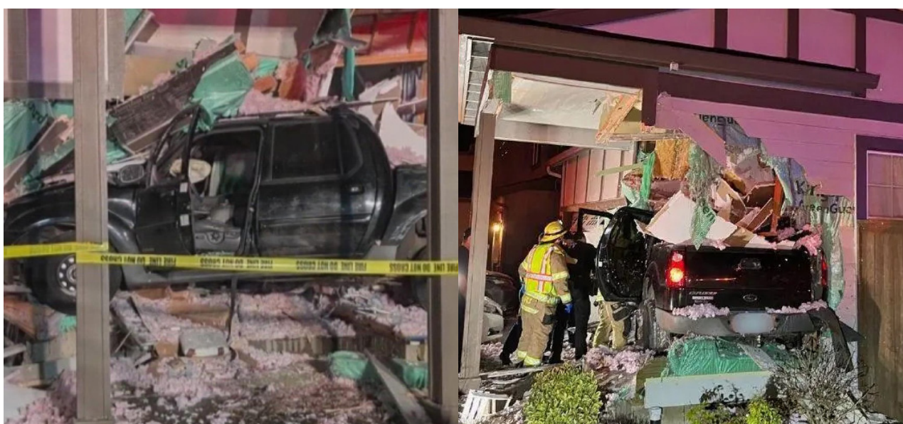
Images of the aftermath of the truck crashing into the Tigard home and first responders responding
